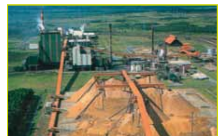
Mondi's pulp and linerboard mill at Richards Bay. Worldwide, Mondi produces 3,8 million tons and Sappi 6,9 million tons of products annually.
